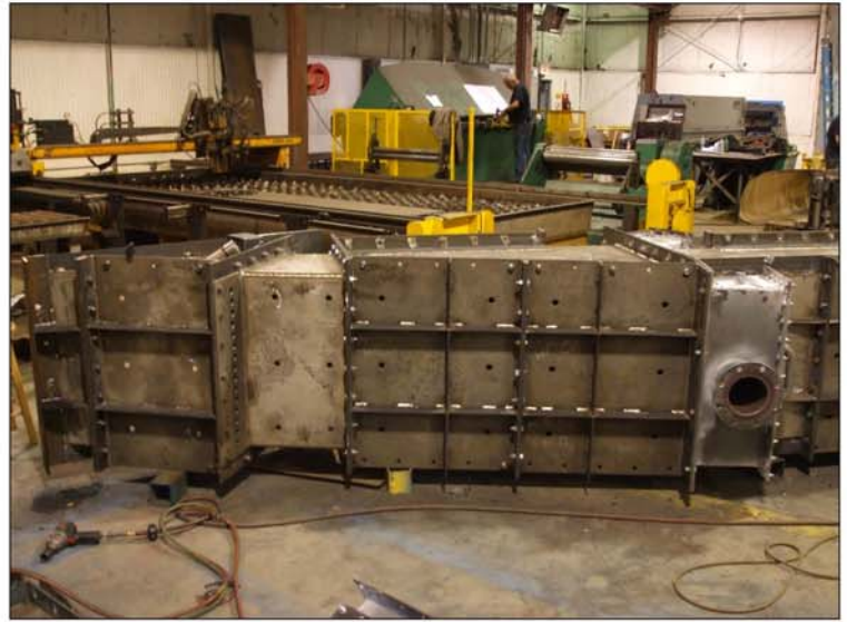
Final welding of chutes completed and trial assembly prior to painting.
